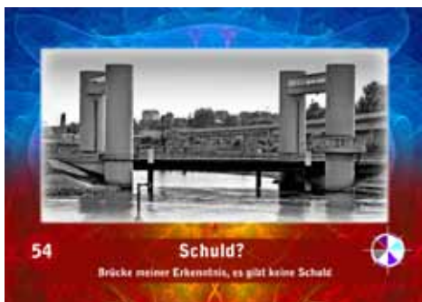
Neckarhubbücke in Mannheim
